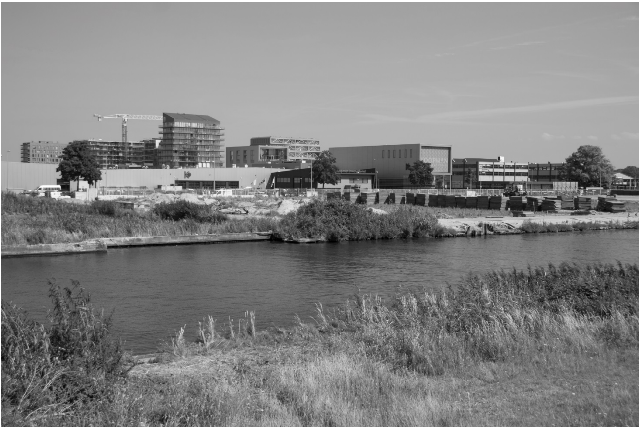
Figure 2 Impression of the Amsterdam Buiksloterham under-construction areas (source: author)
